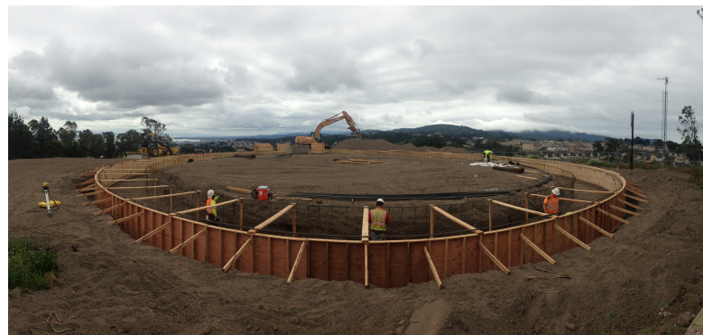
Construction of the North Coast County Water District's Christen Hill Tank, 2015
